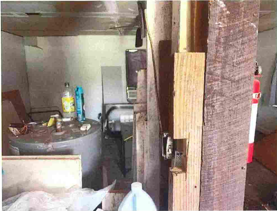
Updated photo taken on June 23, 2026: Walls appear to be in process of being closed in with no open wall inspections, rubbish and debris inside structure causing fire and safety hazards.
