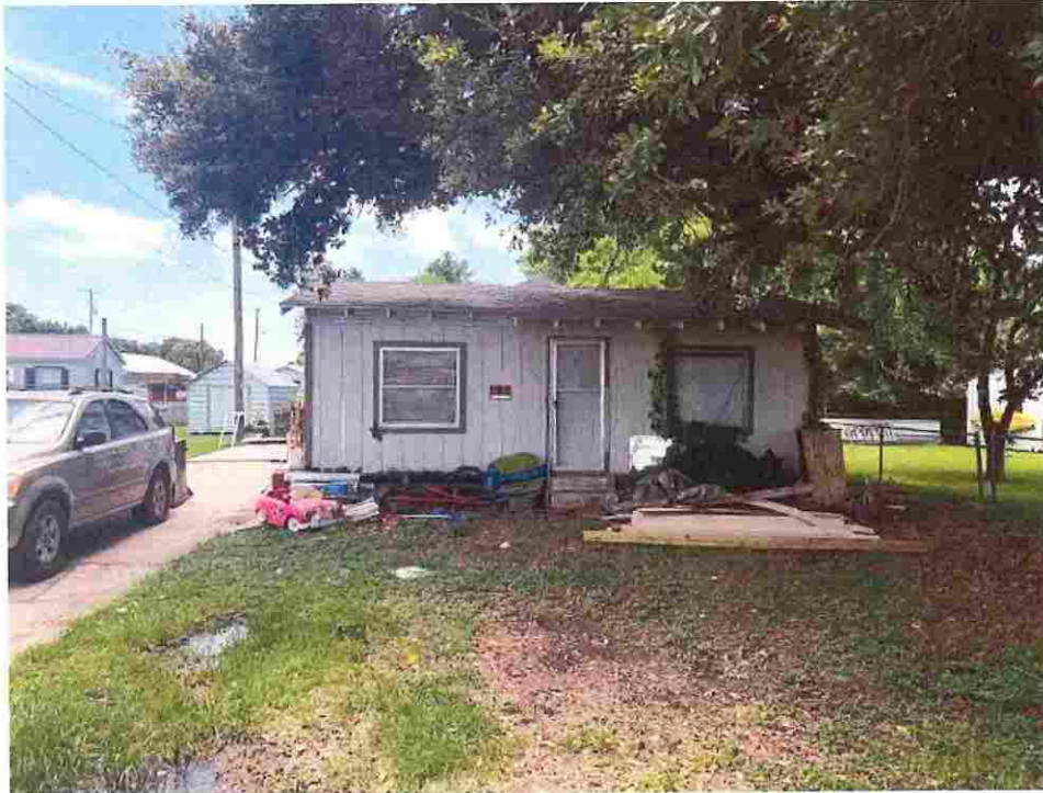
Updated photo taken on June 23, 2026: Structure has continued to deteriorate, foliage growing into structure, rubbish and debris causing blighting.
